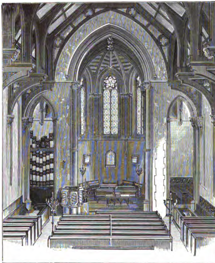
Interior of Clifton Down Congregational Church.
